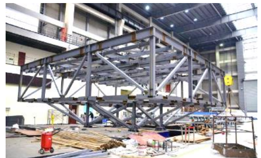
Shaking table test of suspended ceiling
